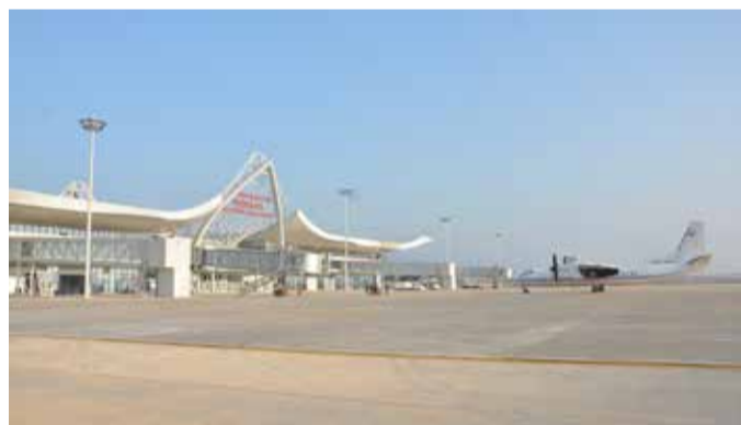
The new international airport in Tonpheung district, Bokeo province.
