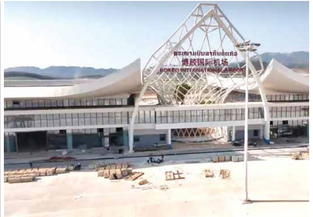
The under-construction terminal at Bokeo international airport.
